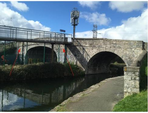
Figure 27 – Existing bridge with engaged piers highlighted.
