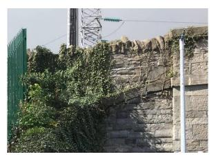
Figure 22 – Original copings visible to south east wing wall.
