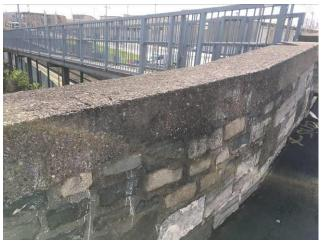
Figure 23 – Poor condition of pointing & concrete copings.
