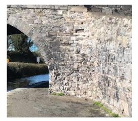
Figure 18 – Weathered facing stone visible, especially below the spring of the arch.
