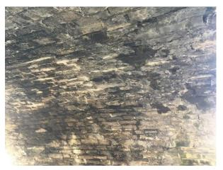
Figure 19 – Condition of canal arch stonework.
