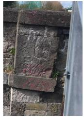
Figure 24 – Pier stone damaged.
