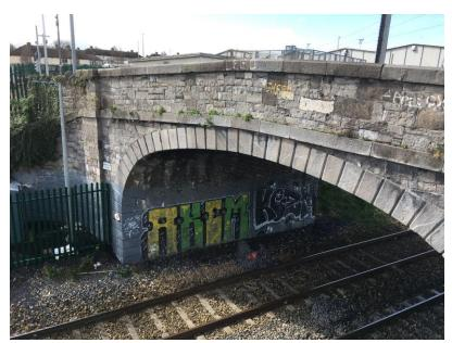
Figure 4 – Railway arch showing voussoirs of arch ring, string course, engaged pier and a wing wall curving away to the east (left hand side).
