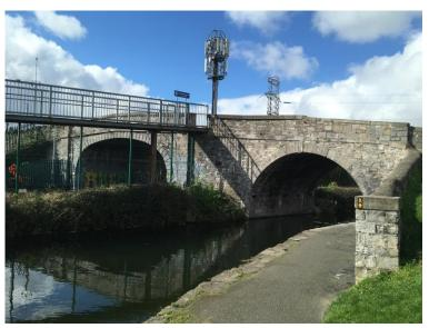
Figure 1 – East elevation of Broome Bridge showing both arches with the railway on the left hand side and canal on the right hand side.
